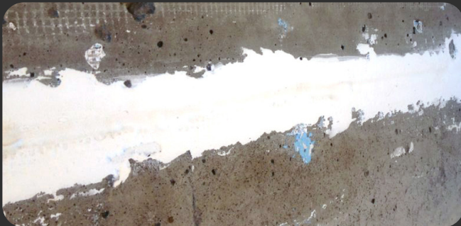
CONCRETE REPAIR AND REMEDIATION
