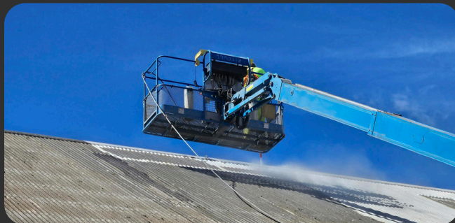
HIGH-RISK AND REMOTE PROJECT DELIVERY
