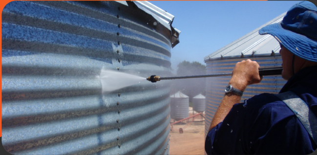
PROTECTIVE COATINGS AND MEMBRANE APPLICATION
